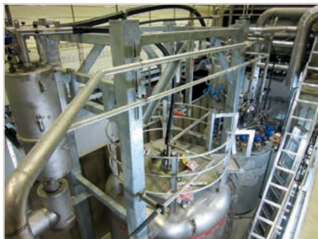
Fig. 7: The liquefier, 7000-L dewar and interconnecting piping in the TPS utility area.
