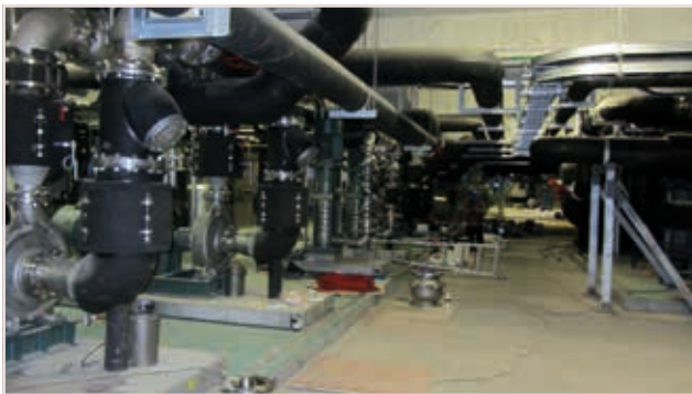
Fig. 4: The main pumping system for circulation of de-ionized water.
