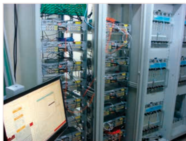
Fig. 10: BPM electronics and corrector power supplies installed at TPS equipment area for testing.
