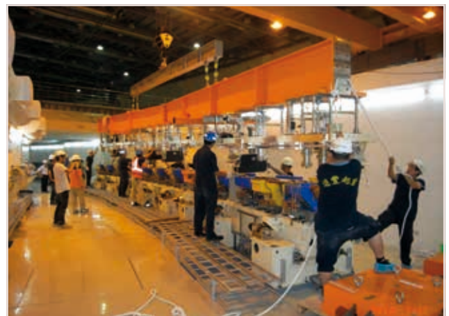
Fig. 5: Installation of a 14-m vacuum cell on the girders.
